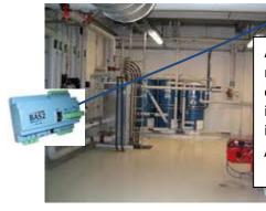
A new controller replaces the often outdated instrumentation in the boiler room / substation.
