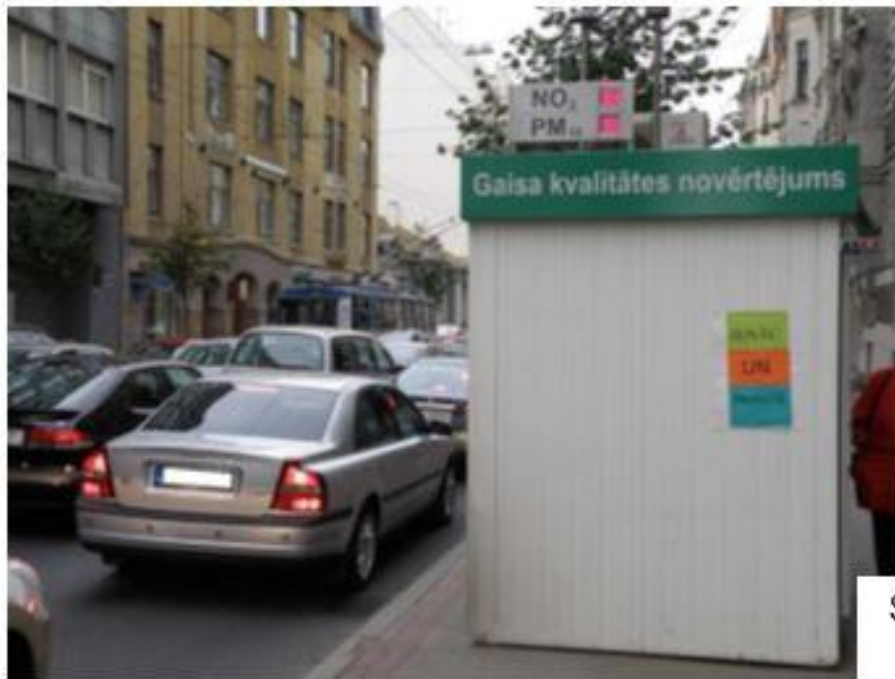
Street canyon on Kr.Valdemāra Street 18 in city centre: multi-instrumental classical point type AQMS
