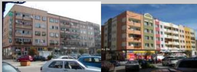
Apartment buildings in Dzierżoniów before and after the thermo insulation.
