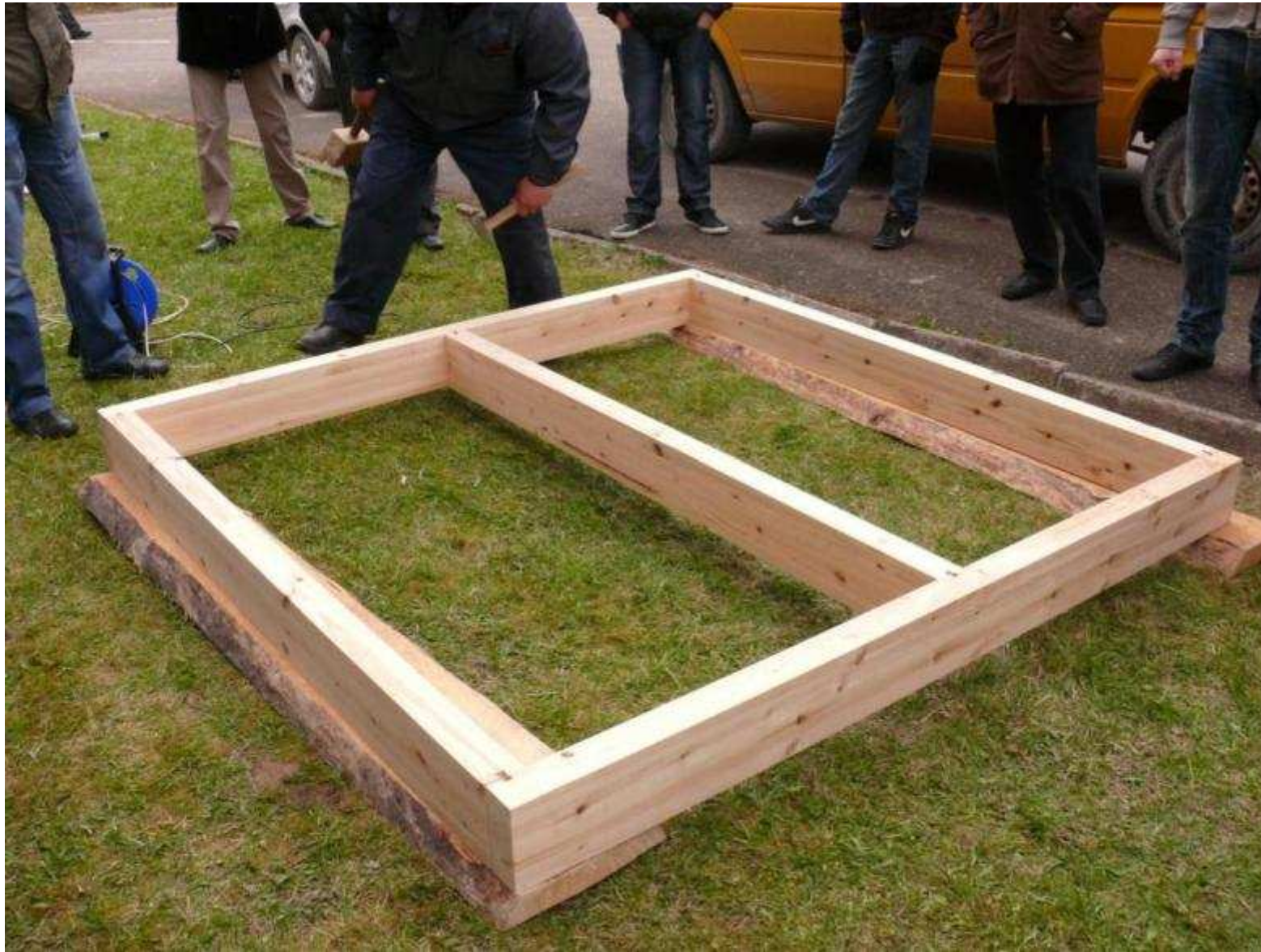
Window mounting frame is assembled
