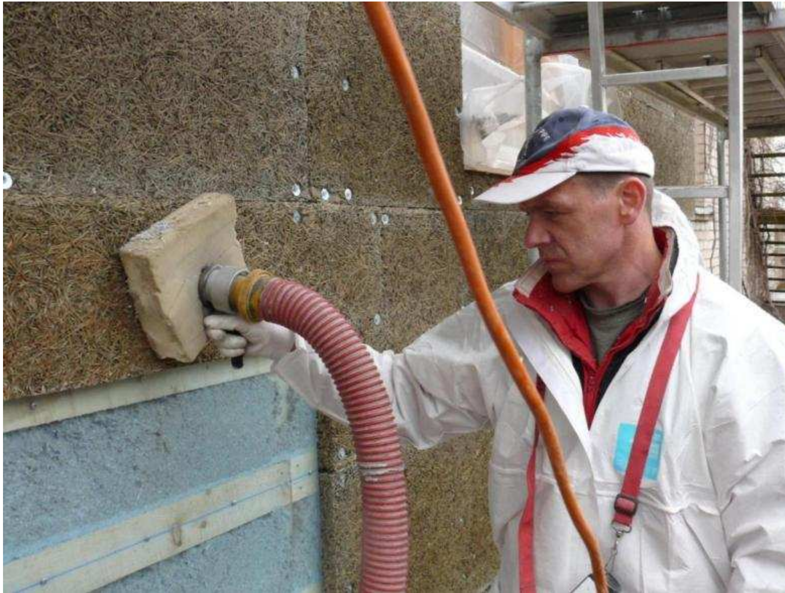
Cellulose blowing
